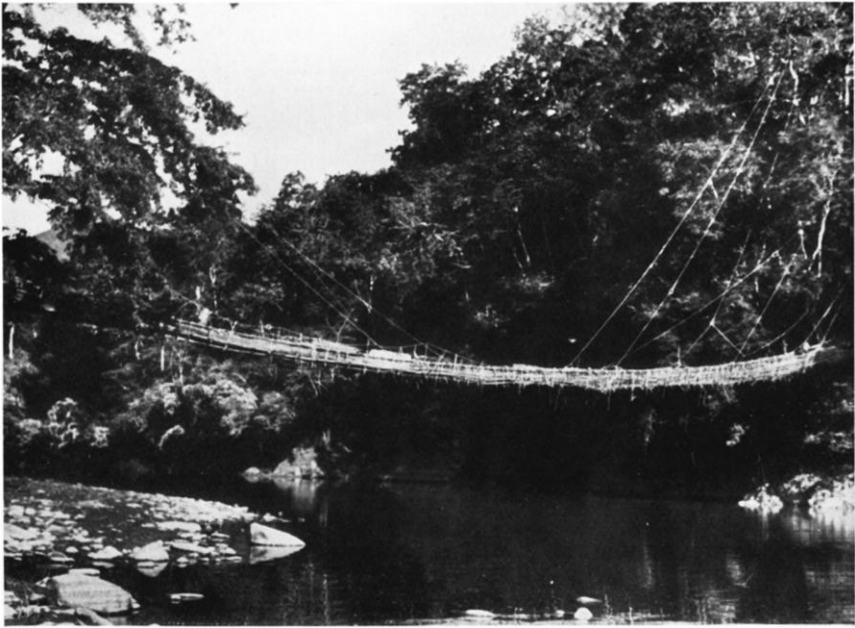
Konyak Naga bridge of suspended cane
